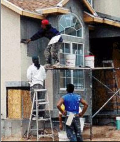
*These workers are not protected from being struck by falling objects because they are working around/under other workers and not wearing hardhats.*
