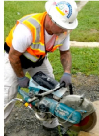
Applying water to the blade of a handheld power saw reduces the amount of dust created when cutting.
